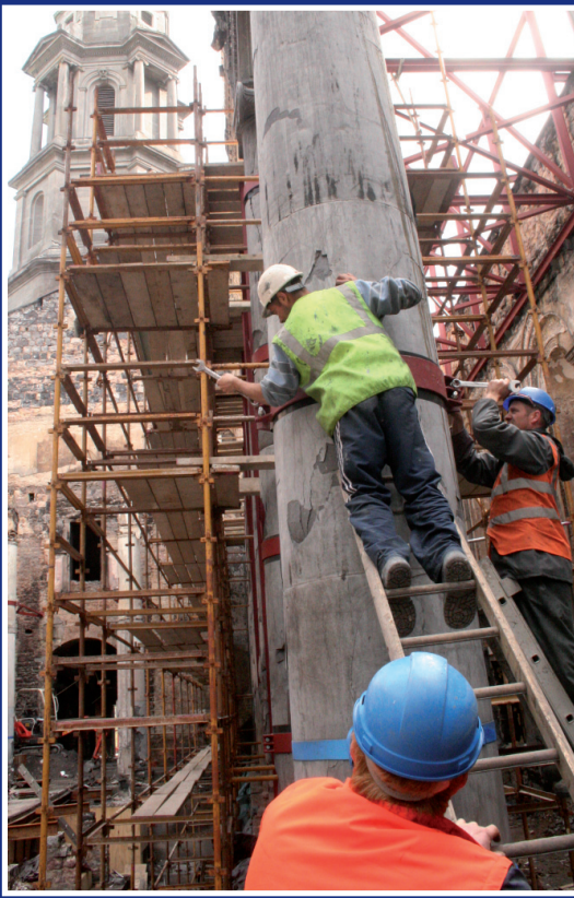
Pillars being secured as part of the emergency works.
