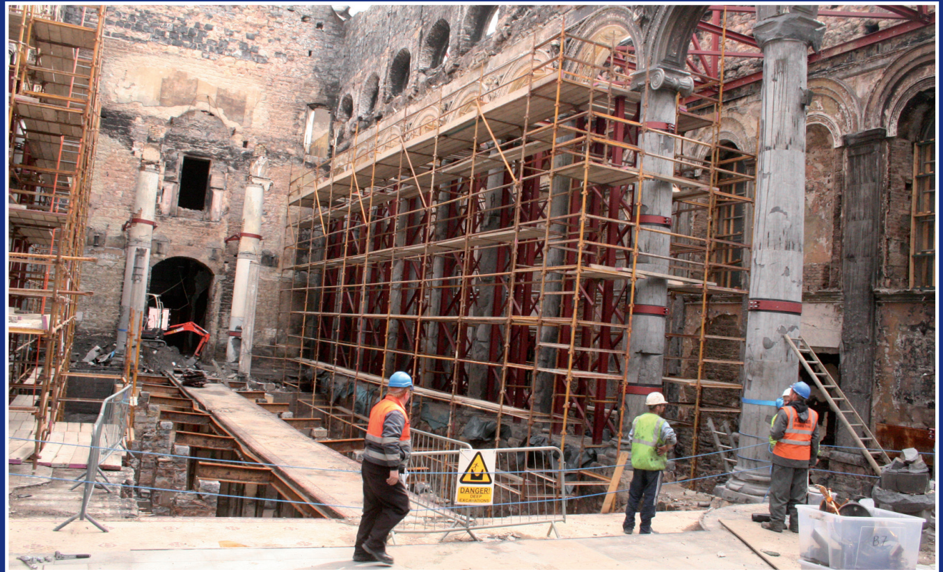
Extensive steelwork is put in place to safeguard the building as part of the emergency works.
