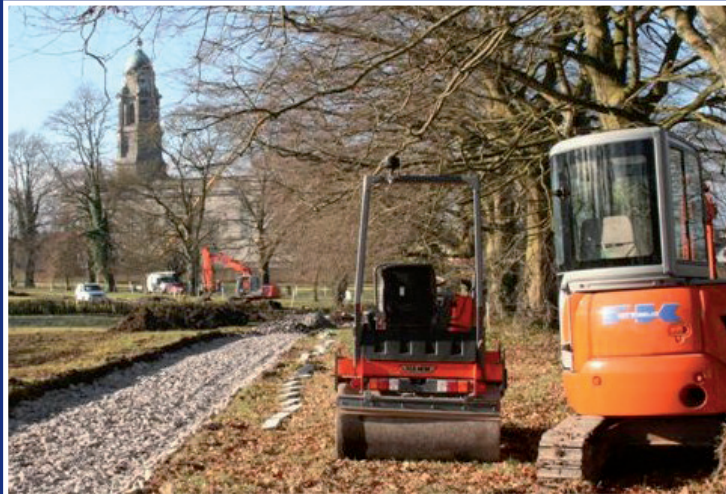
Work on the new pathway begins.
