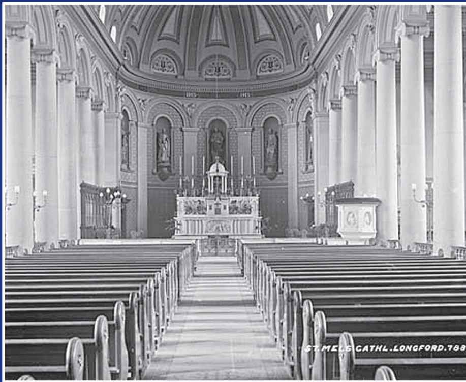
Original interior of St. Mel's Cathedral.
