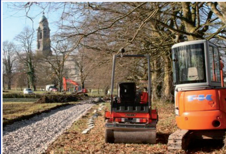
Work on the new pathway begins.
